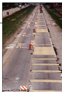
“D” Cracking
